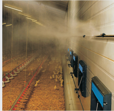
DA 2000 in broiler house
